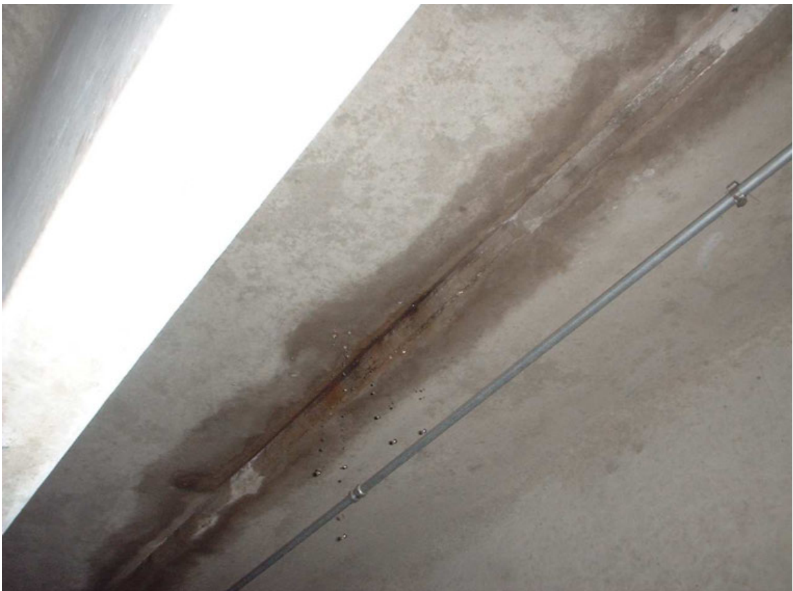
Figure 4-2: Leaking parking deck joint.
