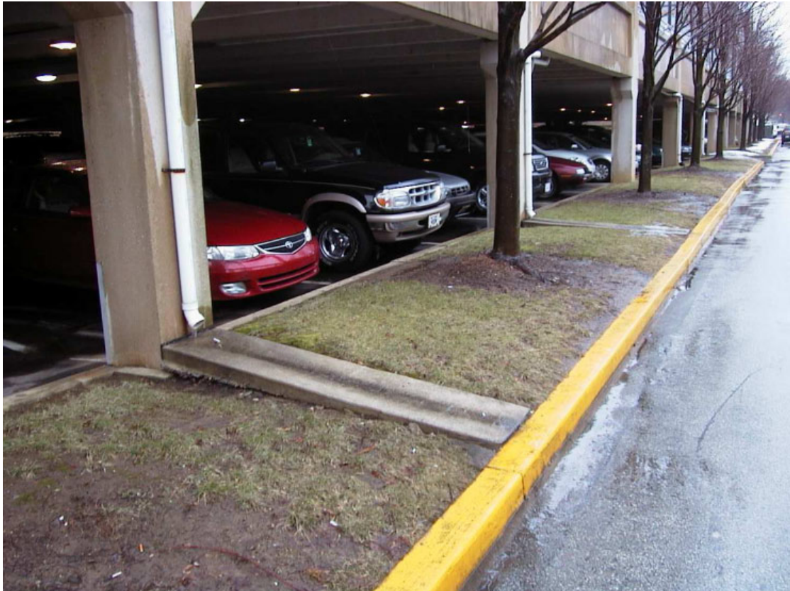
Figure 1-4: PVC downspouts before the trench construction and re-routing.
