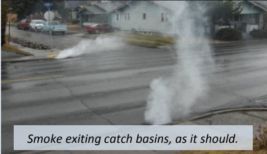
Smoke blown into storm drain manhole.
