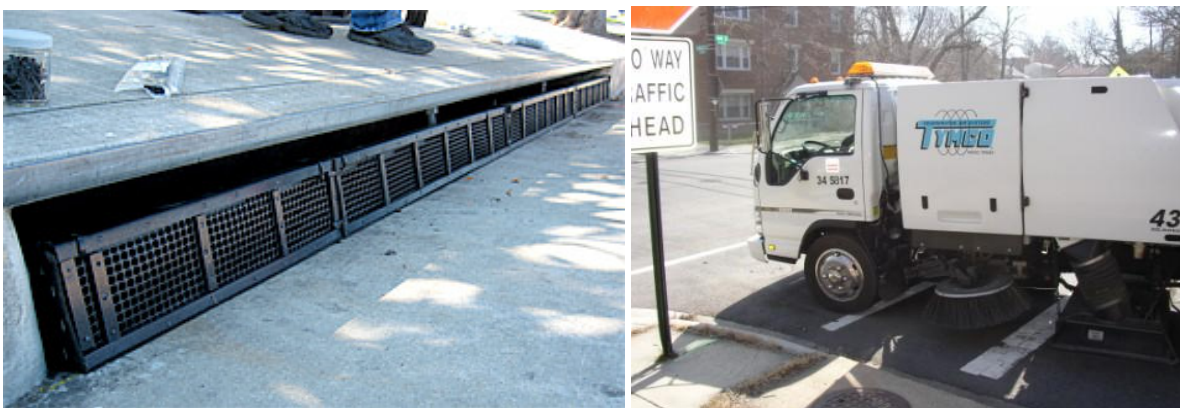
Figure 4.5. Retractable inlet screens and street sweeping are two key strategies recommended to reduce trash (Sources: City of Los Angeles Stormwater Program http://www.lastormwater.org/siteorg/program/poll_abate/cbscreens.htm and Center for Watershed Protection).
