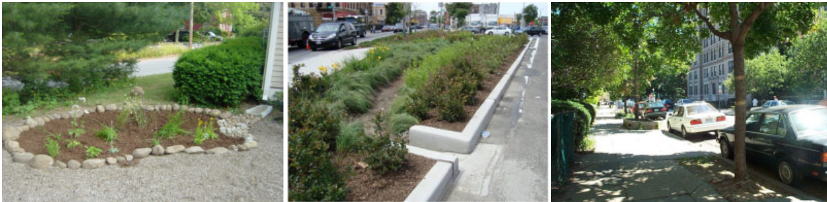
Figure I.5. Urban green infrastructure includes the network of trees, open space and other natural areas that capture rainfall and reduce runoff, thereby protecting water quality. Large mature trees also provide many community benefits, such as shade and cooling, increased property values, and benefits to human health and wellness (Sources: National NEMO Network, New York City Department of Parks and Recreation, Center for Watershed Protection).
