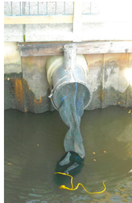
Figure 4.7. Outfall netting devices capture trash from the storm drain system before reaching local waterways (Source: Kristar, Inc.)
