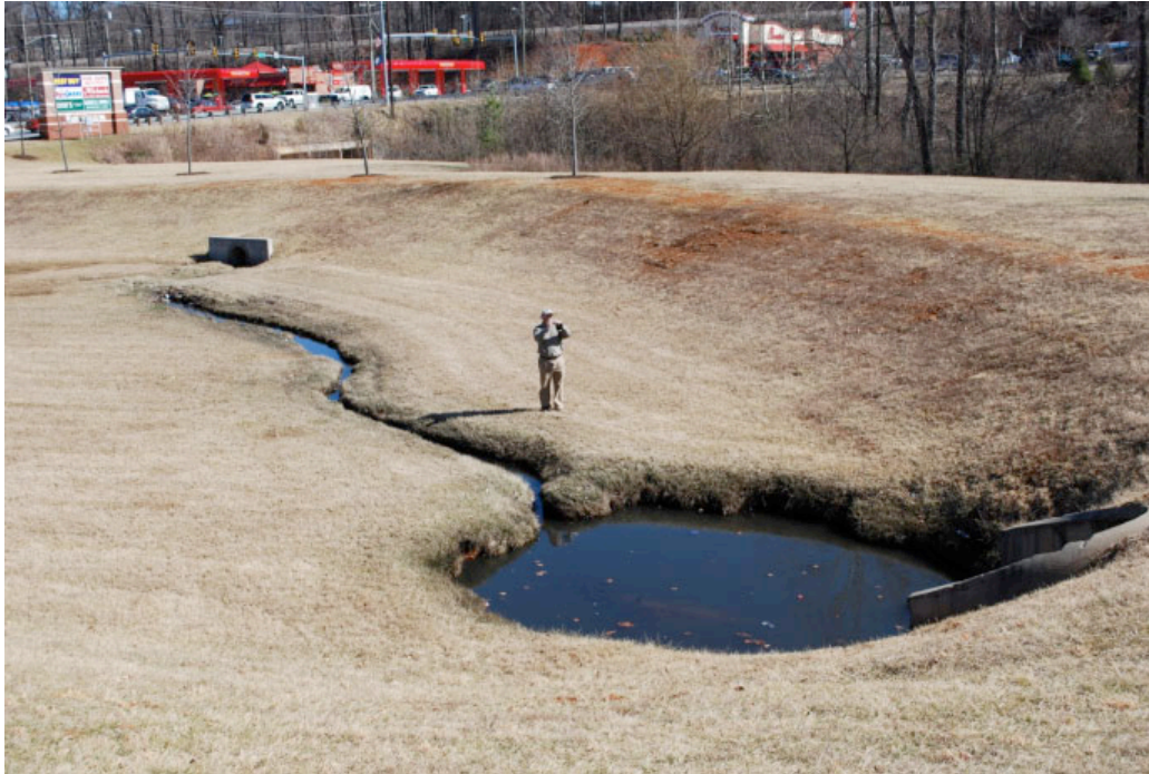
Figure 5.6. This pond could be retrofitted with relatively minor modifications to provide water quality treatment for small storms (Source: Center for Watershed Protection)
