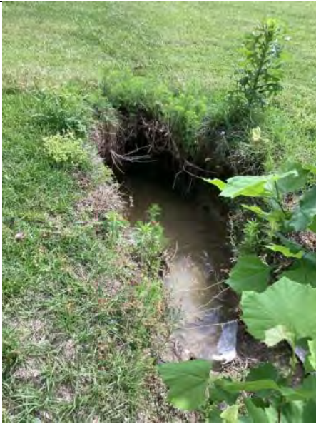
Site 8 – Greenville Fire Dept. Station 5
