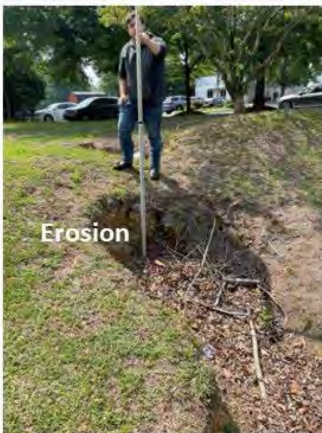
Figure 7. Examples of observed dry detention basin challenges including shallow groundwater, trash deposition, unmaintained vegetation, erosion, and clogged inlets/outlets.
