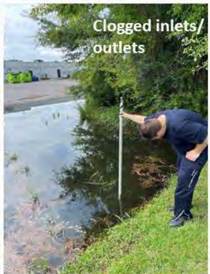
Figure 7. Examples of observed dry detention basin challenges including shallow groundwater, trash deposition, unmaintained vegetation, erosion, and clogged inlets/outlets.
