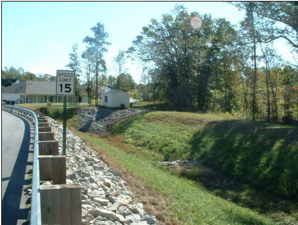
Dry detention basin. Source: http://www.colonial-heights.com/assets/images/009.jpg
