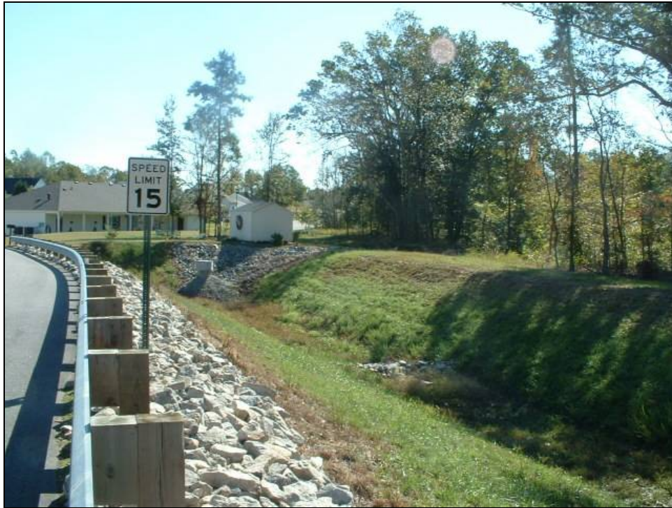
Dry detention basin. Source: http://www.colonial-heights.com/assets/images/009.jpg
