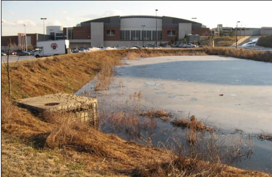
Wet pond receiving stormwater runoff from parking lots serving the Comcast Center sports arena and other facilities at the University of Maryland, College Park. Emergent wetland vegetation (cattails and other species) is visible in shallow waters along the shoreline. Photo by A.H. Baldwin.
