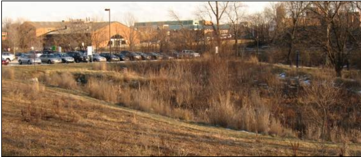
Stormwater wetland at the University of Maryland, College Park. Runoff from the parking lot enters the wetland from the left, flows in a roughly U-shaped counterclockwise pattern, and discharges via a riser at the top center of the wetland. Photo by A.H. Baldwin.
