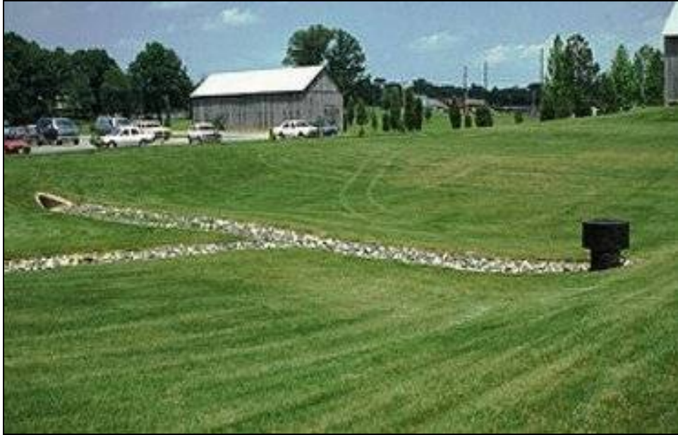
Dry detention pond with grass surface. Source: Chesapeake Bay Program 2006
