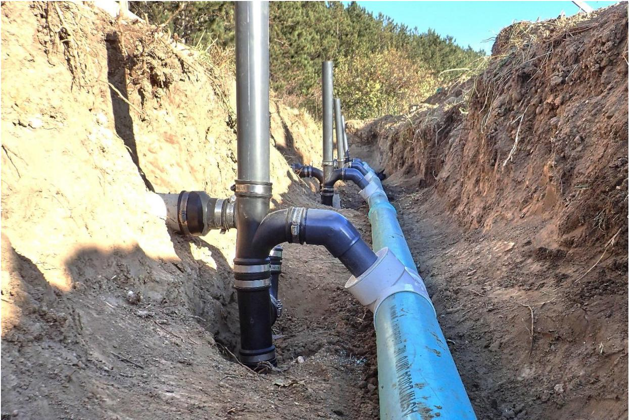
**Figure 9: Installation of traps for housing conductivity sensors.**
