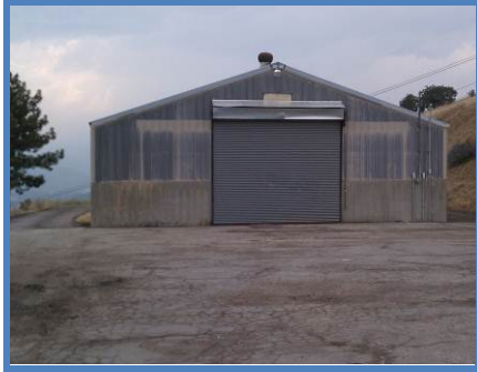
District 8 – CalTrans Hilt Storage
