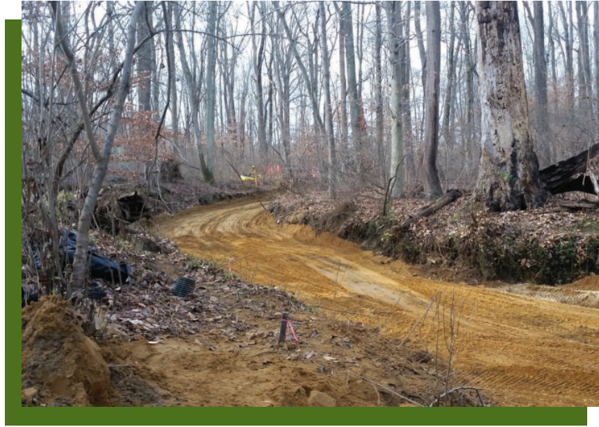
Figure 14. RSC sand and woodchip haul road constructed in-stream to raise the stream bottom and to minimize impacts to the riparian area (Source: MD DNR RSC Construction Guidance ; Photo Credit: Underwood & Associates, Inc., and Actaeon Group)
