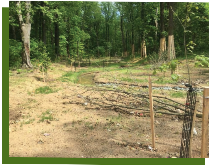
Figure 7. Tree planking around existing trees prevents damage during stream restoration construction (Source: Ecotone, Inc.)
