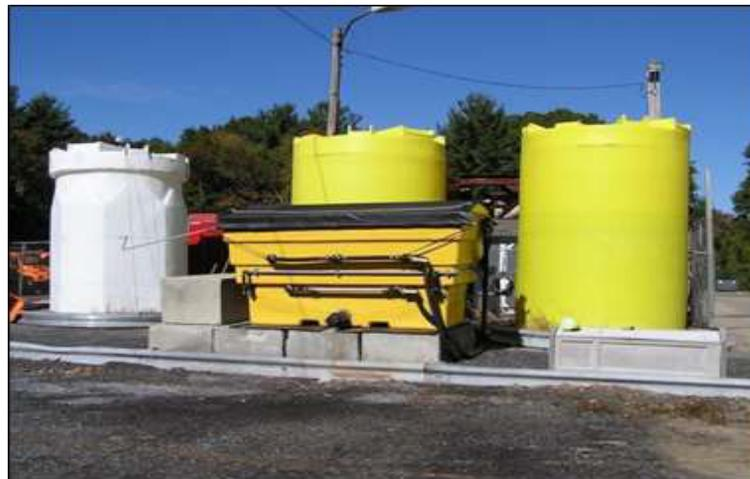
Figure 6: Brine Mixing (Sodium Chloride) and Storage (Sodium Chloride and Magnesium Chloride) Tanks, Putnam Garage
