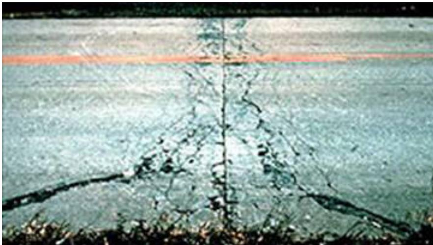
FIGURE 6.6. MODERATE SEVERITY DURABILITY "D" CRACKING (PHOTO FROM [92])
