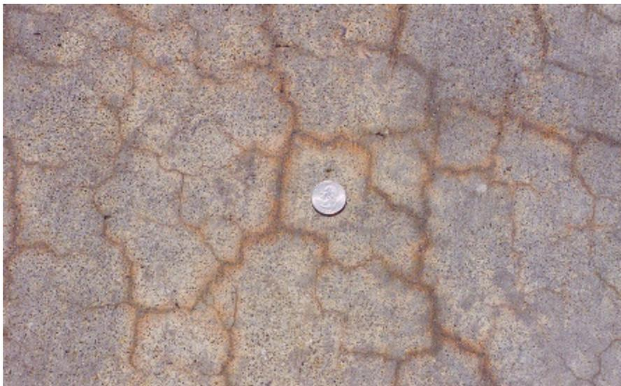
FIGURE 6.3. PORTLAND CEMENT CONCRETE SURFACE MAP CRACKING (PHOTO FROM [92])
