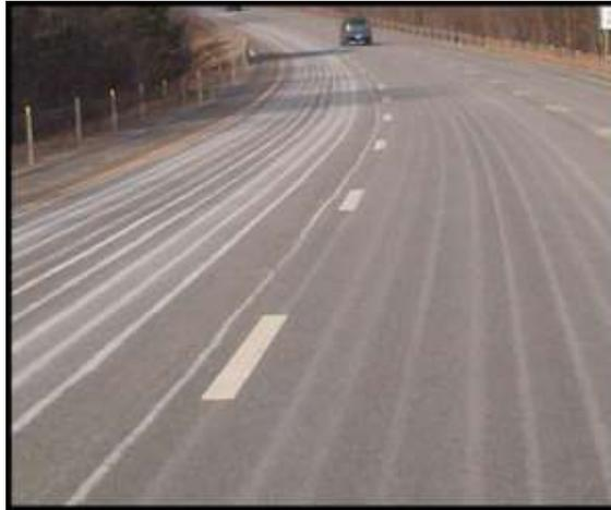
Figure 5: Pavement Pre-Treated with Sodium Chloride Brine Solution
