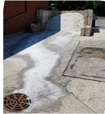
No "rivers of salt" should be leaving the storage area.
