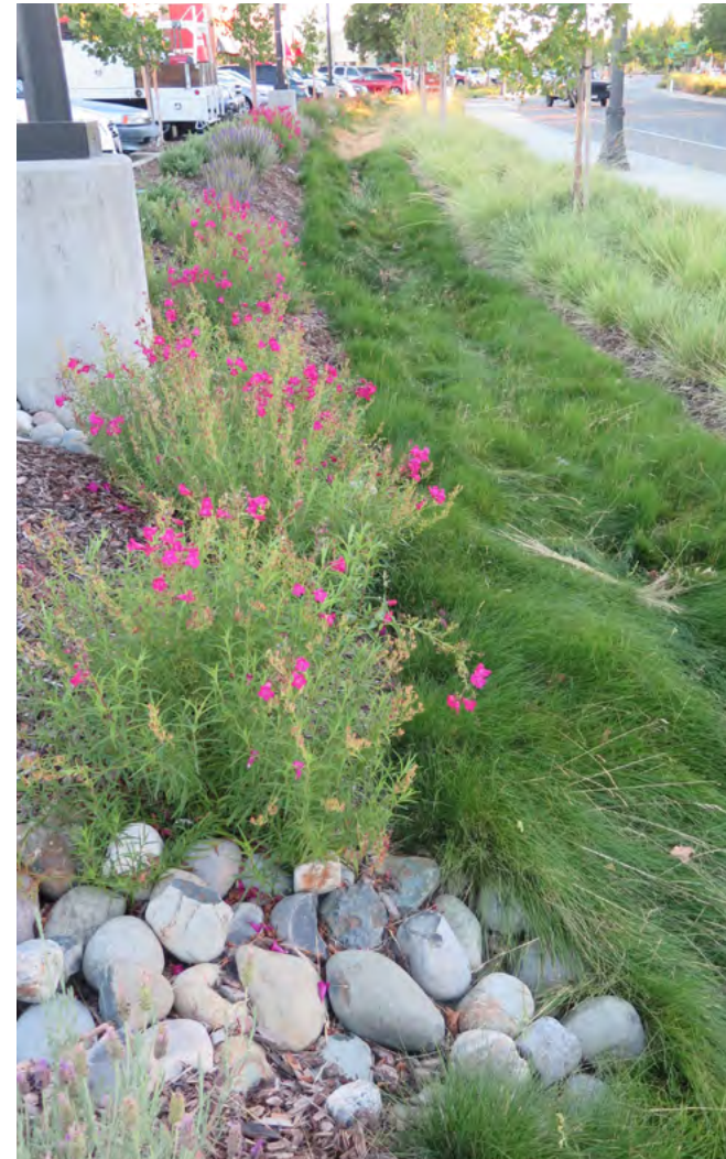
Stormwater runoff from a parking lot is directed to a vegetated swale via cobblestone inlets, managing stormwater while also enhancing public space. Photo: Krystal Zamora
