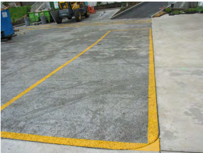
Pervious asphalt in Portland, OR. Photo: Rosey Jencks
