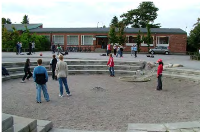
A dry detention pond sited within a Children's play space in Augustenborg, Malmö/Sweden tests different methods of reducing and detaining peak stormwater flows while enhancing the neighborhood. Photo: Sharon Danks
