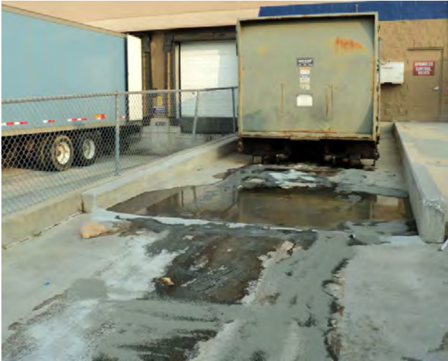
Loading docks are another source of stormwater pollutants. Photo: Stormwaterjess
