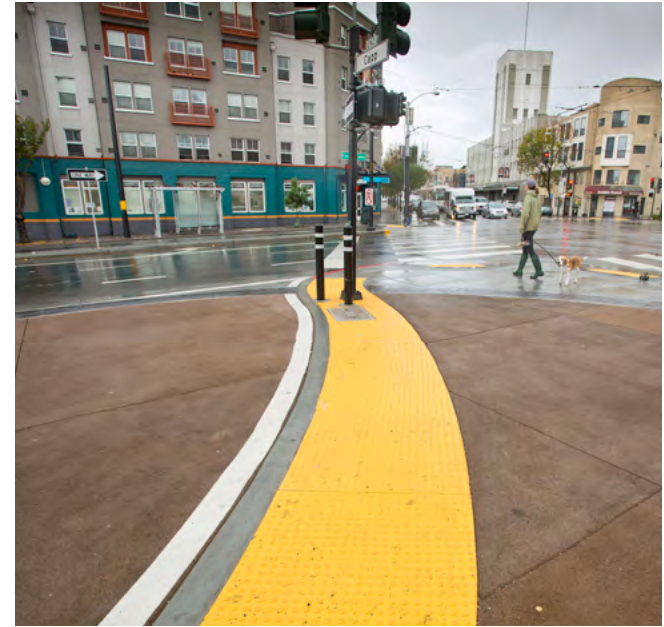
Permeable concrete installed as part of the Cesar Chavez Streetscape Improvement Project in San Francisco, CA. Photo: Robin Scheswhol
