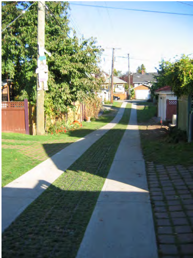
“Country Lanes” in Vancouver, British Columbia enhance the alley’s aesthetic quality and reduce stormwater discharge to the City’s stormsewer system by allowing runoff to flow over vegetation and infiltrate into the ground. Photo: Rosey Jencks
