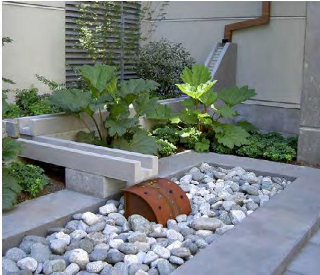
This infiltration trench doubles as stormwater art in Portland, OR. Photo: Ken Kortkamp
