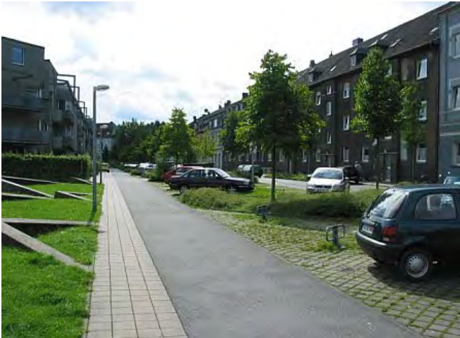
Permeable pavers are used in parking spaces in Germany. Photo: Rosey Jencks
