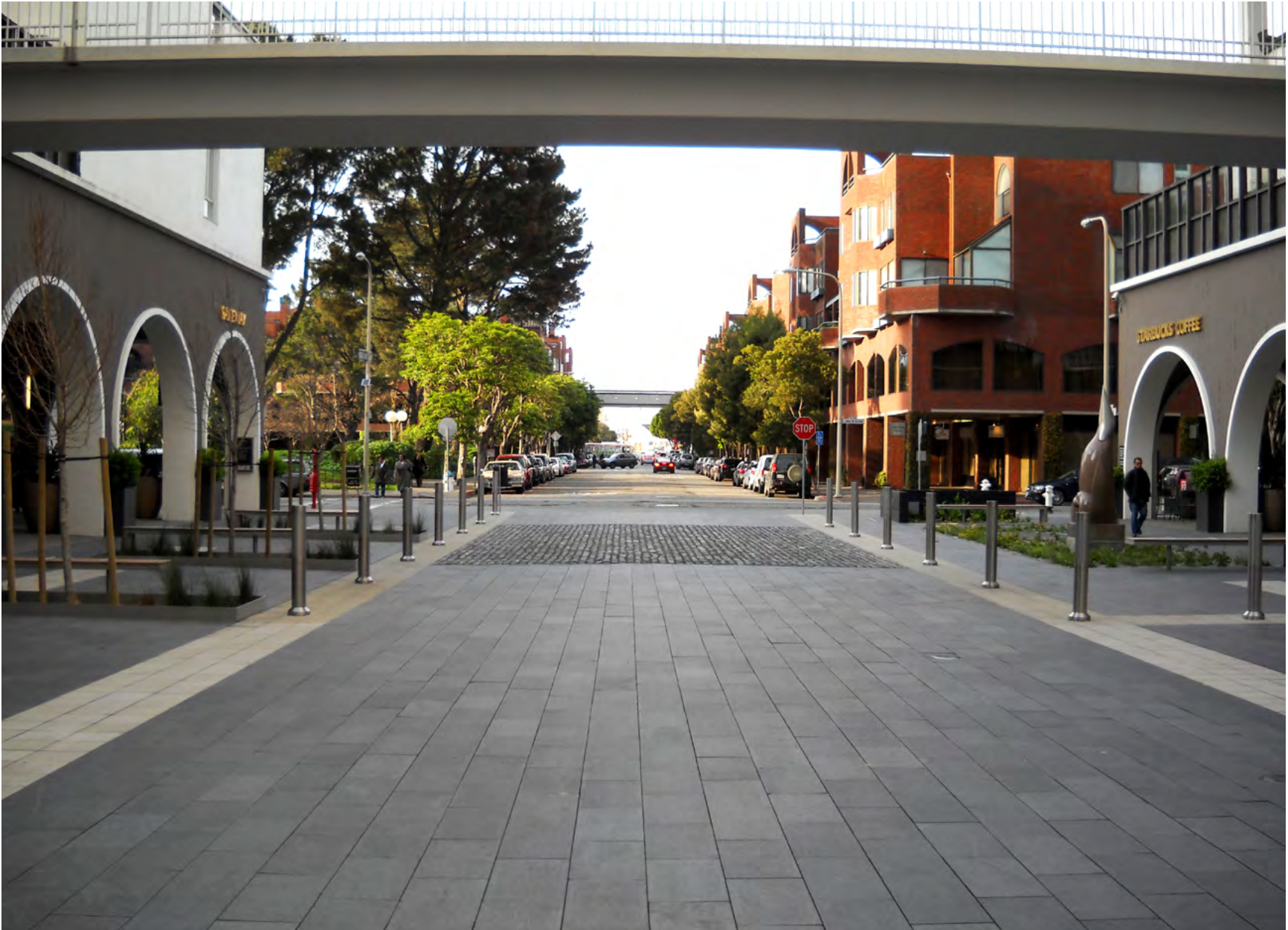
This plaza features permeable paving and bioretention in San Francisco, CA. Photo: Sherwood Design Engineers
