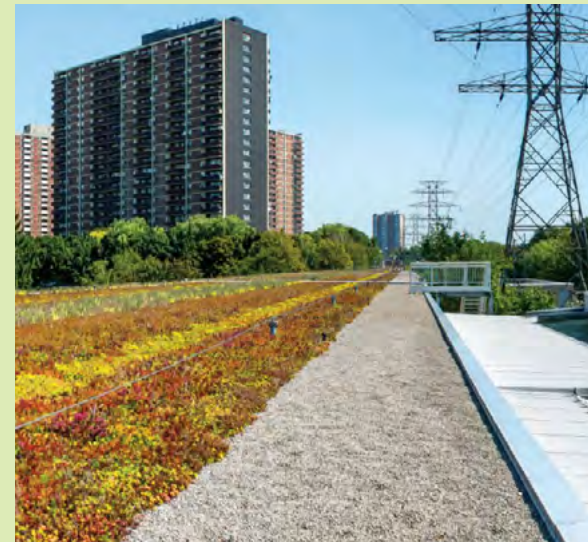
An extensive living roof atop a Subway Station in Toronto. Photo: City of Toronto
