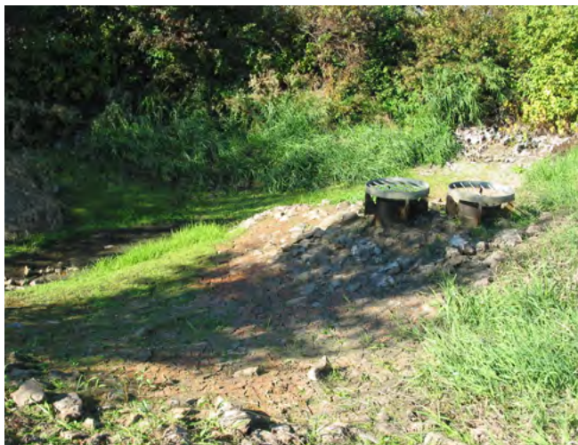
An infiltration basin in Waterworks Gardens at the King County East Division Reclamation Plant, Renton, WA, is part of an environmental art park that treats stormwater. Runoff flows through stormwater treatment ponds, and the wetlands form an earth/water sculpture that funnels, captures and releases water. Photo: Rosey Jencks
