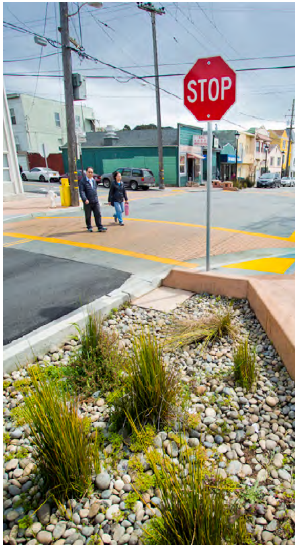
Leland Avenue in San Francisco features permeable paving and bioretention in the right-of-way. Photo: Robin Scheswhol
