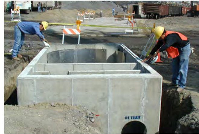
Swirl separators remove grit and debris from stormwater runoff. Photo: Contech
