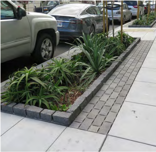
Permeable pavement surrounding planters in the public right-of-way in San Francisco, CA. Photo: Krystal Zamora
