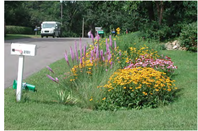
Residential rain garden in Maplewood, MN captures and infiltrates runoff from both residential yard and the street. Photo: City of Maplewood
