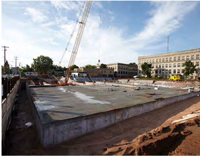
Construction of an underground stormwater detention basin beneath the City Hall parking lot in downtown Oshkosh, Wisconsin. Photo: Precast-Prestressed Concrete Institute
