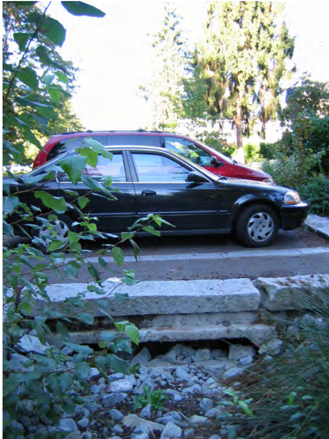
This infiltration trench doubles as a parking strip along the Sustainable Streetscapes and Fish Habitat Enhancement Project: Crown Street, Vancouver, British Columbia. Photo: Rosey Jencks
