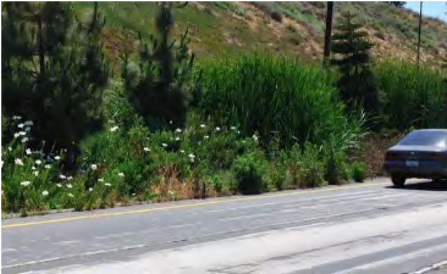
This vegetated buffer strip along the Imperial Highway in Los Angeles, CA slows stormwater runoff from the highway. Photo: LA Stormwater Program
