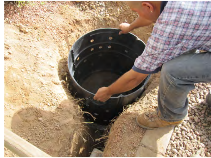
Installation of a pre-cast drywell, note the holes to allow stormwater infiltration. Photo: Lake George Association
