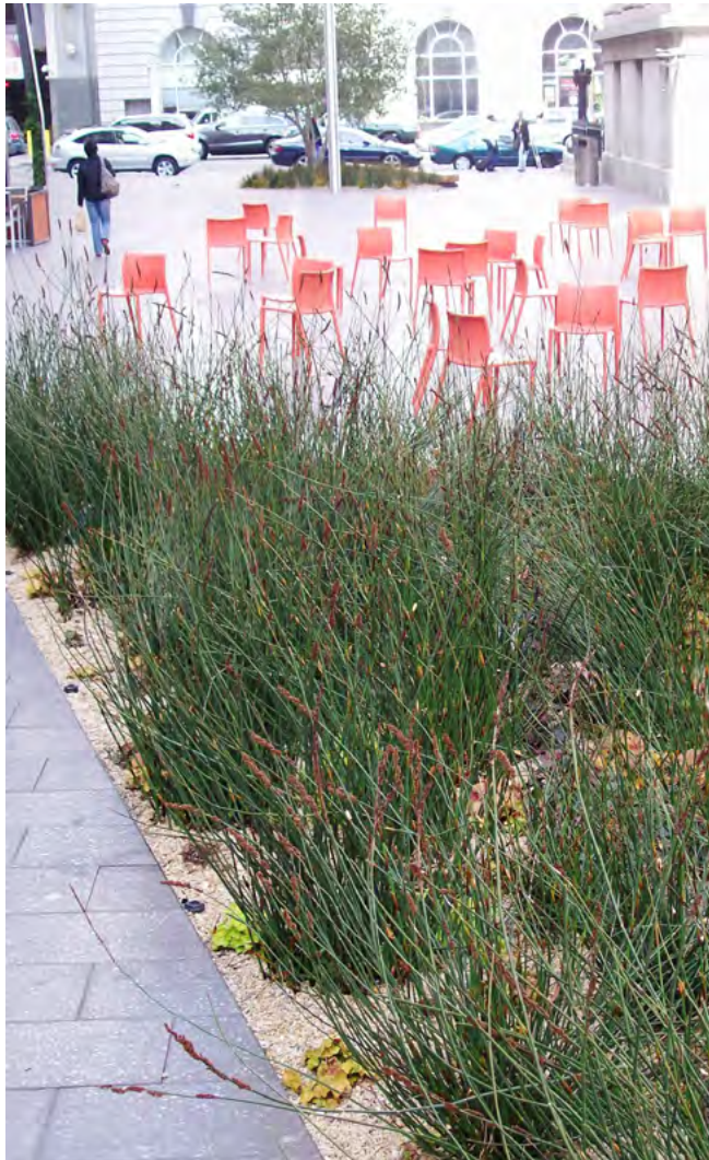
A rain garden captures and infiltrates stormwater from the paved surface in Mint Plaza, San Francisco. Photo: Rosey Jencks
