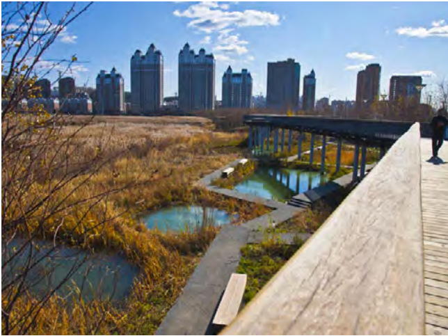
Constructed wetlands not only create a park-like settings, but they also remove contaminants from stormwater and provide flood control. Photo: Programmed Property Services
