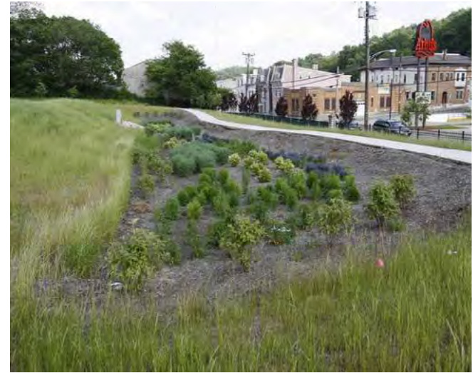
An infiltration basin at the Saint Francis Court Apartments in South Fairmount, Cincinnati is used to reduce the volume of stormwater that enters the sewer system. Photo: Gary Landers
