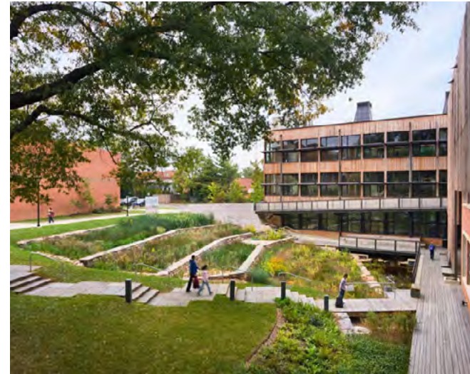
This project's constructed wetland treats the building's wastewater on-site while the pond and rain garden prevent stormwater runoff. Photo: Albert Vecerka
