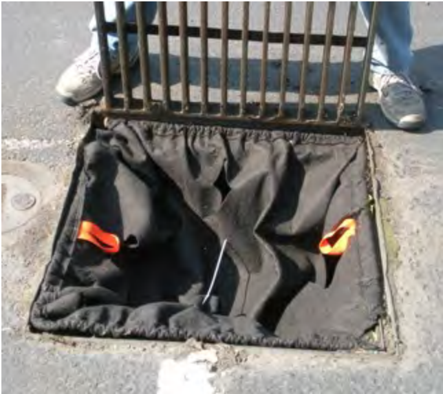
Drain insert in a stormwater catch basin. Photo: EnviroMet
