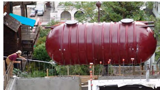
Installation of a cistern in Sausalito, CA. Photo: Sherwood Engineers
