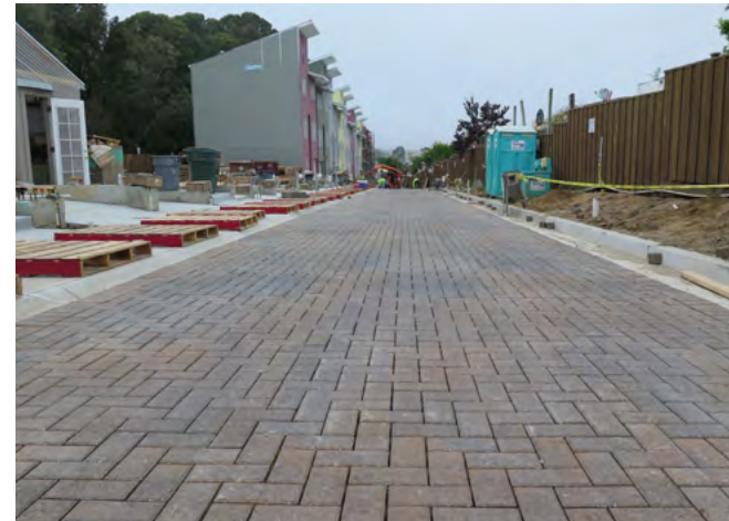
This Habitat for Humanity construction project features curb-to-curb permeable paving along a private residential road. Photo: Krystal Zamora
