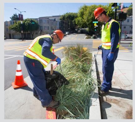
Set up safety perimeter, wear a hard hat and safety vest, and use a rake or grabbers to remove trash and debris from the planter.
