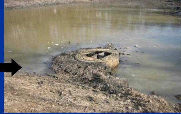
Beaver Lodges that Block Primary Outlet Works
