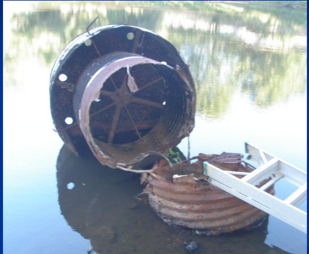
Deteriorated/Rusted Risers
