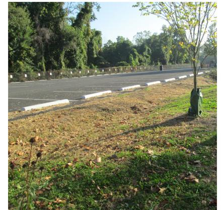
Figure 1-14. Examples of Stormwater Swales
