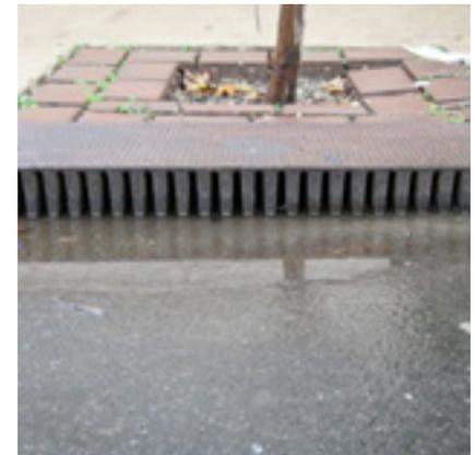
Figure 1-18. Examples of Stormwater Trees in Philadelphia
