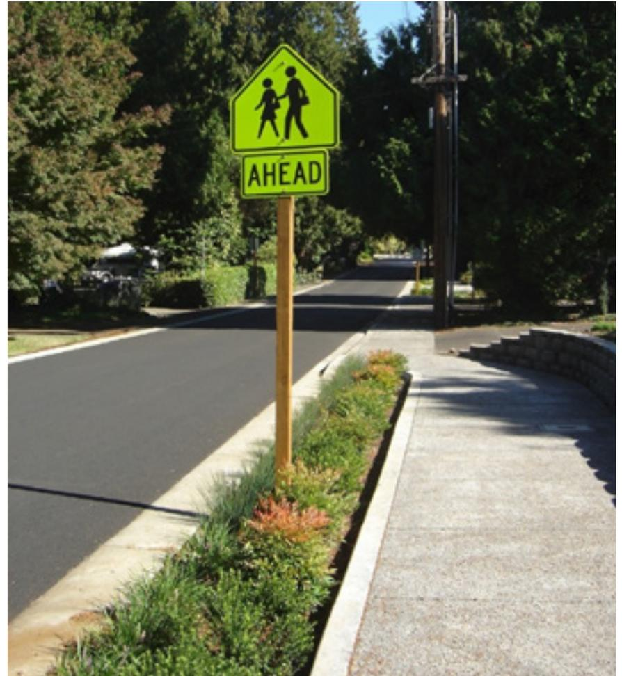
Figure 1-28. Example of a Green Gutter in Portland, Oregon
