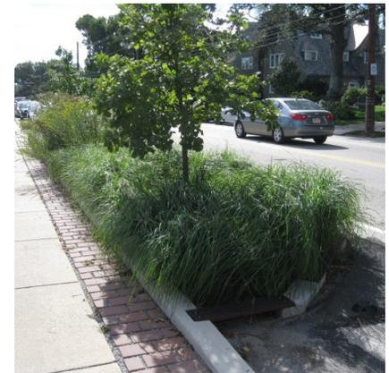
Figure 1-7. Examples of Stormwater Bump-outs in Philadelphia
