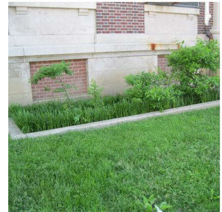
Figure 1-5. Examples of Stormwater Planters in Philadelphia
