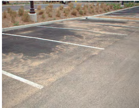
Figure 8-1 Porous asphalt pavement clogged by runoff sediments from an unstabilized adjacent area, Philadelphia, PA
