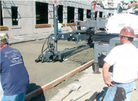
Figure 3-21 Industrial loading dock. Finishing performed with a pervious concrete laser screed, Lacey, WA Source: Puget Sound Concrete Specification Council
