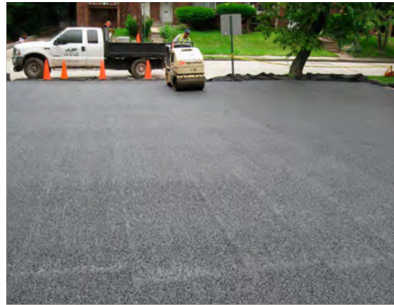
Figure 2-21 A small roller smooths seams of porous asphalt surface course, Yeadon, PA
