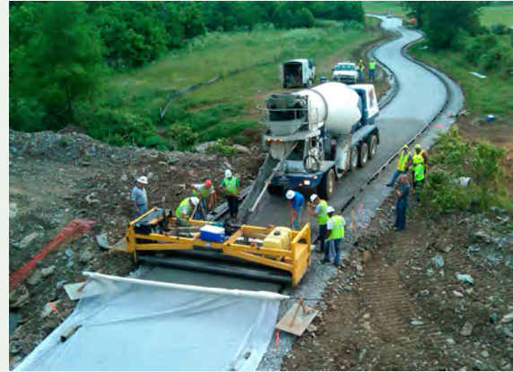
Figure 3-20 Finishing performed with a power-roller screed, Legacy Recreational Trail, Lexington, KY Source: Concrete Promotional Group, Inc.
