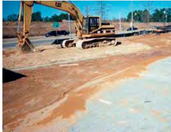
Figure 3-23 Erosion and sediment control failure, GA Source: WR Grace
