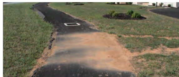
Figure 2-22 Sediment-laden stormwater runoff clogs the porous asphalt, Campbelltown, PA
