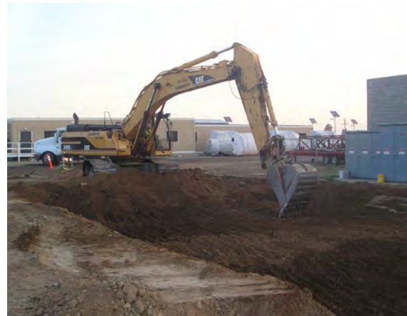
Figure 2-15 Excavator operating from outside the excavation to prevent compaction of subgrade, Modesto, CA
