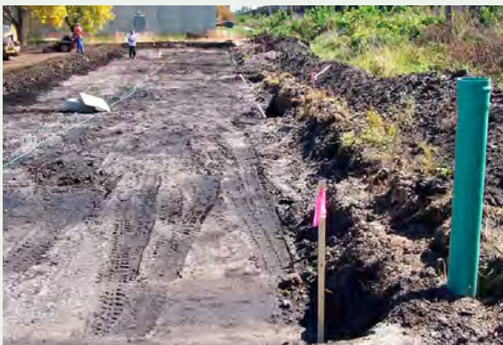
Figure 3-15 Excavation of base for aggregate storage layer prior to scarification and placement of geotextile fabric, Ames, IA
