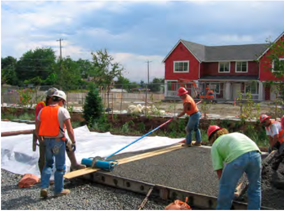
Figure 7-5 Installation of this pervious concrete roadway takes careful planning, High Point Redevelopment Phase 1, Seattle, WA
