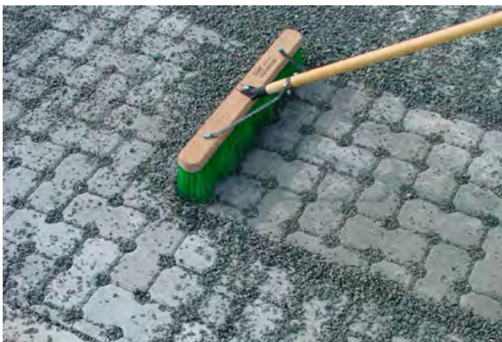
Figure 8-16 Replacement is simple and done with a broom or with mechanical sweepers for larger areas. Source: NCSU
