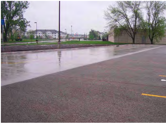
Figure 3-4 Pervious concrete adjacent to traditional concrete during a rainfall, Ames, IA Source: John Kevern
