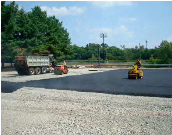
Figure 2-14 Porous asphalt installation, Peabody, MA
