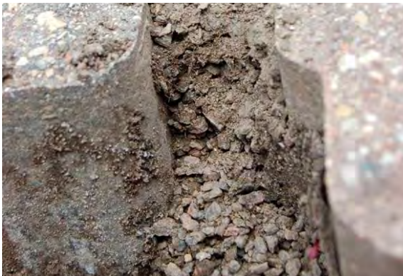
Figure 8-14 PICP opening showing trapped sediment at the top with aggregate under it Source: NCSU
