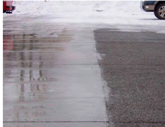
Figure 3-14 Standard concrete adjacent to pervious concrete in cold climate, Iowa State University, Ames, IA
