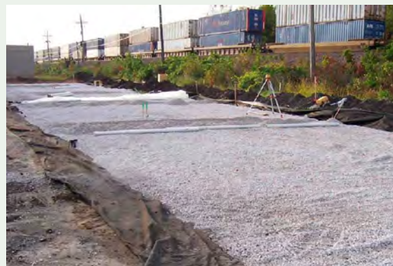
Figure 3-16 Aggregate base after installation of geotextile fabric, Ames, IA
