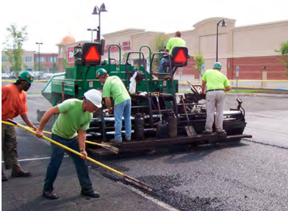
Figure 2-20 Installation of porous asphalt over the aggregate base layer with a tracked paver, Warrington, PA
