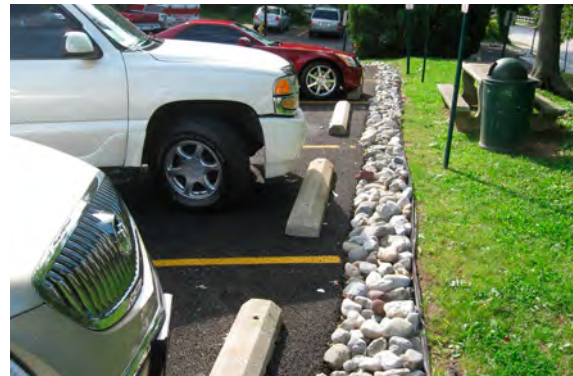
Figure 2-13 River stone edge offers a backup method for runoff to enter the reservoir course, Yeadon, PA Source: CH2M HILL
