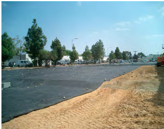
Figure 2-16 Earthen berms and geotextile, San Diego, CA
