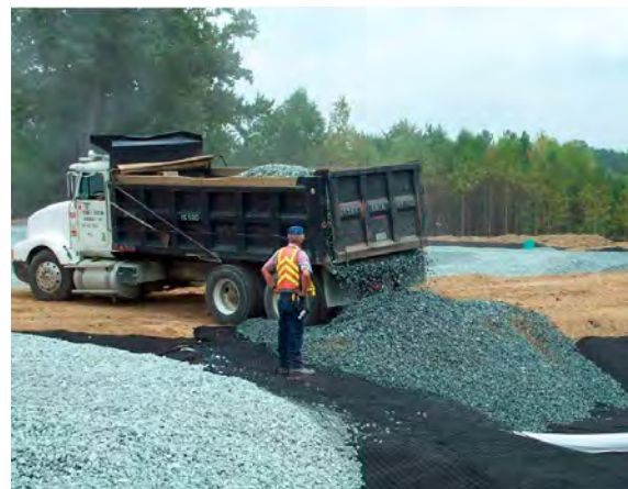
Figure 2-19 Aggregate placed in the bed from the edge to prevent compaction, Chapel Hill, NC
