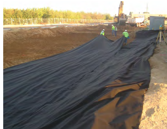
Figure 2-17 Geotextile being placed by hand to avoid compaction of subgrade, Modesto, CA
