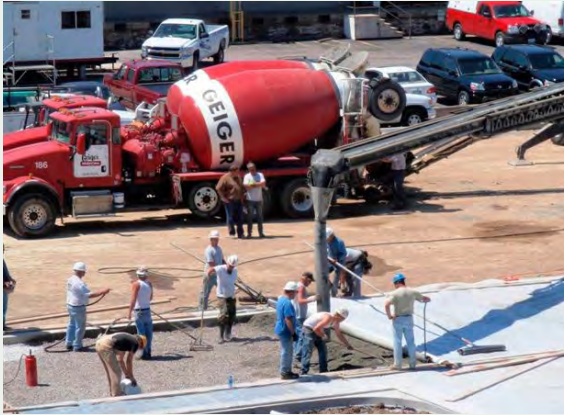
Figure 3-19 Concrete deposited as close as possible to the final location. Finishing performed with a hydraulic roller screed, Overland Park, KS Source: Concrete Promotional Group, Inc.
