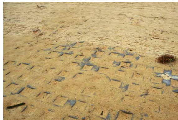
Figure 8-17 Hollowed out concrete grid pavement voids penetrated by mechanical sweeper bristles, leaving loose sand from large voids on pavement surface to be swept back into voids. Source: NCSU
