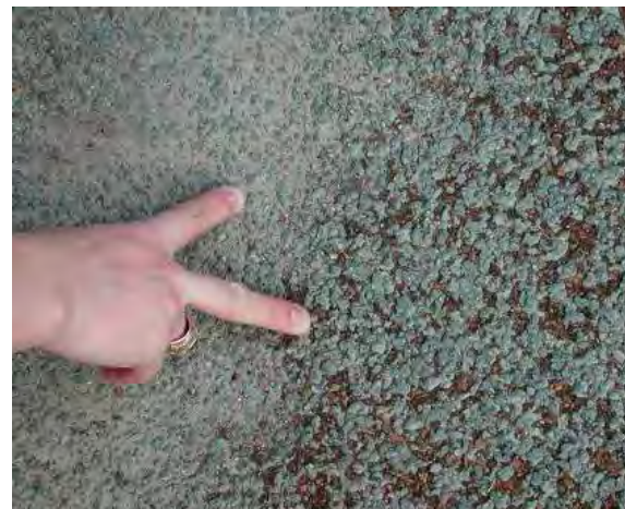
Figure 8-6 Visual inspection of a pervious concrete lot shows sediment and leaf debris accumulation
