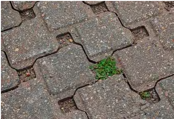
Figure 8-12 Before vacuum cleaning of a PICP parking lot surface that was not cleaned for seven years Source: ICPI
