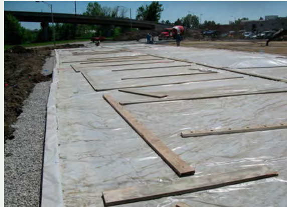
Figure 3-22 Plastic sheeting secured on the pervious concrete, Overland Park, KS Source: Concrete Promotional Group, Inc.
