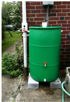
Top-left and bottom-left photos: Rain barrels in use in the City of Lancaster (Source: LiveGREEN)
