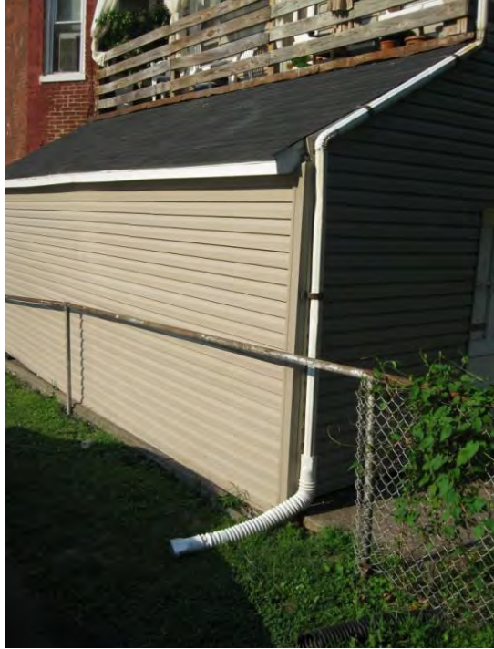
Residential downspout disconnection in Lancaster, PA
