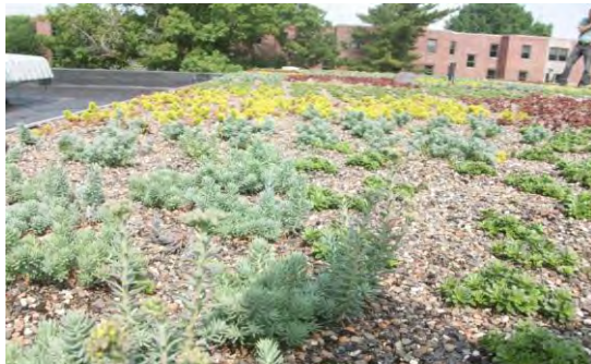
Vegetated Roof at F&M College in Lancaster, PA (Source: LiveGREEN)
