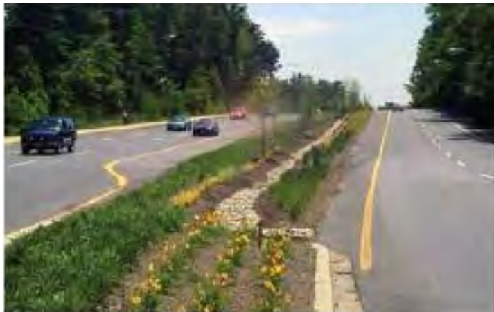
Linear bioretention area along roadway Source: Low Impact Development Center, Inc.
