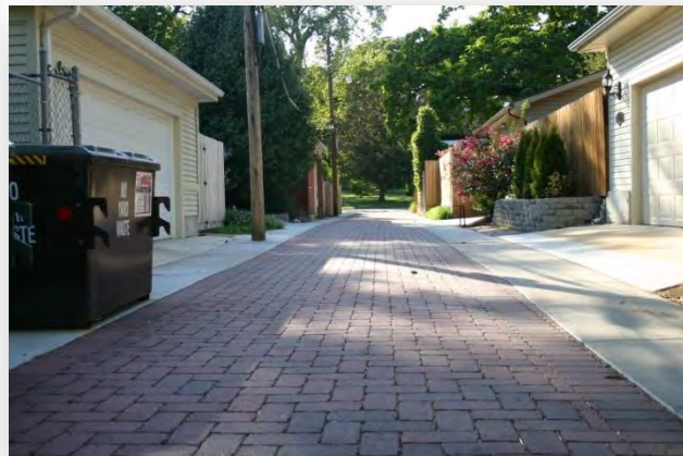
Geyer Porous Paver Alley, St. Louis, MO
