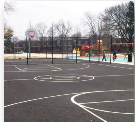
The 6th Ward Park porous basketball court provides runoff reduction at 1/2 the cost of separate grey controls, while also providing community improvements
