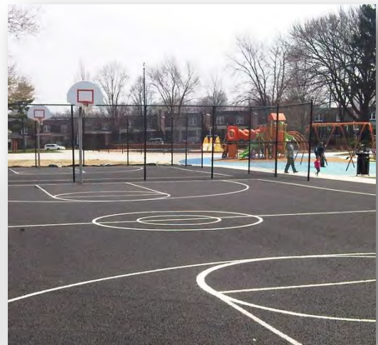
A porous basketball court at 6 th Ward Park plan progressed from idea, to concept, to construction during the development of the GI Plan.
