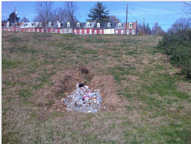
Existing Parking lot connected to grassed swale and outflow to open field.
