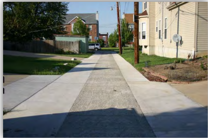
Green Alley with Porous Concrete in St Louis, MO
