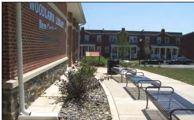
Infiltration planter box at Woodlawn Library, Wilmington, DE
