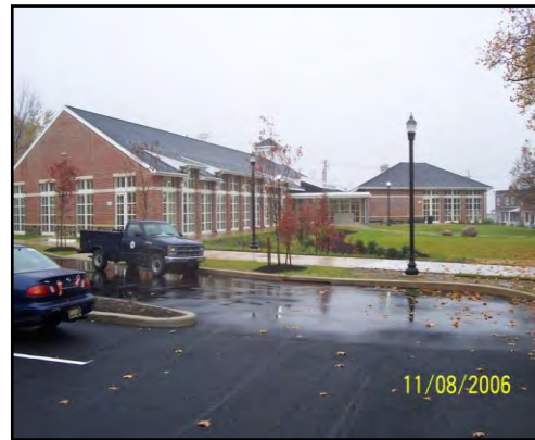
Porous asphalt parking lot in Wilm., DE
