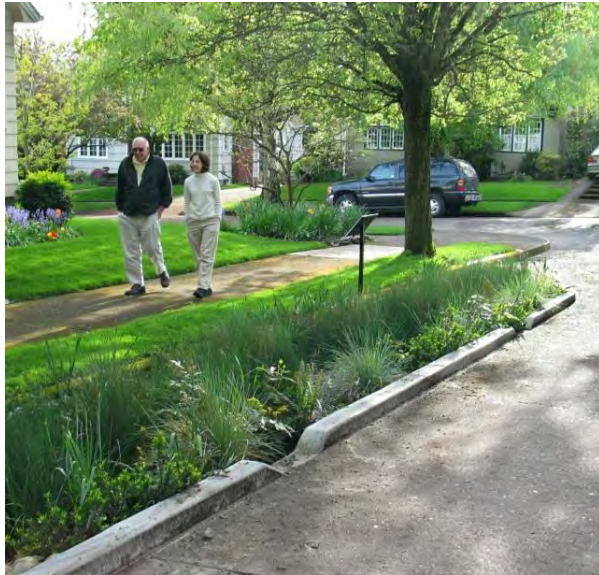
Urban application of a vegetated curb extension in Portland, Oregon (Source: www.artfulstormwater.net )
