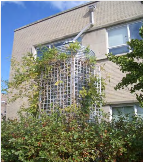
Cistern with Green wall at Chicago Center for Green Technology
