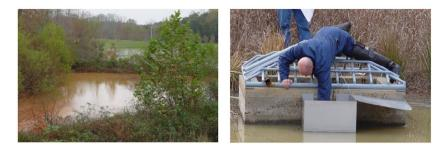
Figure 16. Wet ponds with (left) a forebay and (right) a low flow drawdown structure that have very difficult accessibility in North Carolina, USA.
