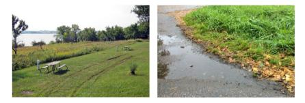
Figure 13. Rutting in soggy soil due to poorly timed mowing/ trimming of turf grass. Flush curb without set-down due to turf growth and sediment accumulation leading to water ponding and sediment accumulation on the road surface.
