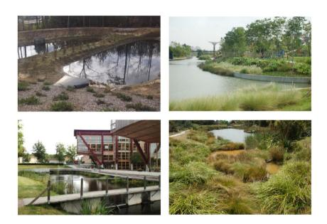
Figure 1. Example wet ponds in North Carolina, USA (with forebay in foreground), Singapore, New Zealand, and Sweden (clockwise from top left).
