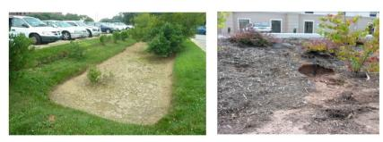
Figure 6. A clogged bioretention cell (left) with an example of internal erosion (right).
