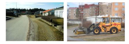
Figure 7. Left: Infiltration trench covered with concrete grid pavers along a residential road in Sweden. An apparent clogging risk due to sand applied during winter maintenance is present. Right: Sediment removal from (*inter alia*) infiltration trenches and buffers strips.
