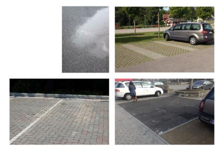
Figure 10. Several examples of permeable pavement types in Connecticut, Sweden, Denmark, and Illinois (clockwise from top left).
