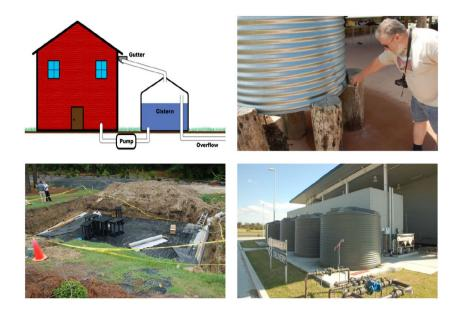
Figure 14. Top left: Rainwater harvesting schematic. Top right and lower right: Above ground rainwater harvesting tanks in New Zealand and Australia. Bottom left: Below ground rainwater harvesting system in North Carolina, USA.
