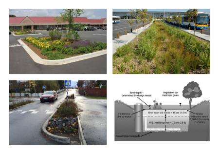
Figure 5. Bioretention cells in North Carolina (top left), Australia (top right) and Sweden (the latter with a small sediment forebay, bottom left) and a cross section of bioretention.
