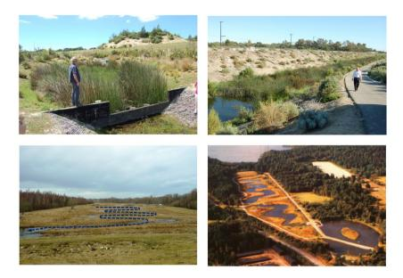
Figure 3. Example wetlands in New Zealand (from outlet structure), California (forebay to left) and Sweden (with sinuous flowpath). Bottom right photo: courtesy of Växjö municipality.
