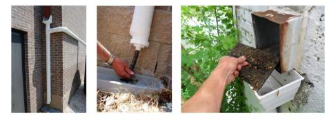
Figure 15. A first flush diverter (left) with clean out (middle). Cleaning out a debris screen (right).
