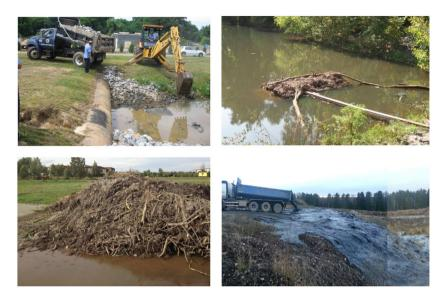
Figure 2. Common wet pond maintenance needs. Top left to right: forebay excavation; outlet/overflow clogging. Bottom left to right: Storage of sediment in the vicinity of the pond which is a risk for leaching of metals during de-watering/drying; disposal of dredged sediment at a landfill in Sweden.
