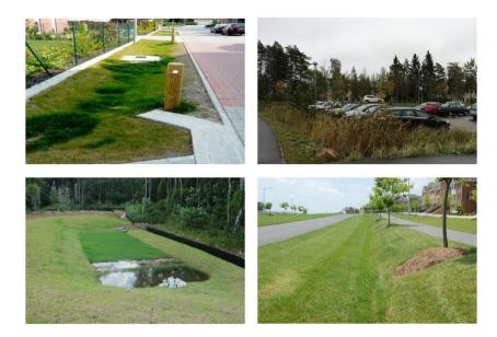
Figure 12. (clockwise from top left) Example swales in Germany, Sweden and Maryland, USA. A filter strip in North Carolina, USA.
