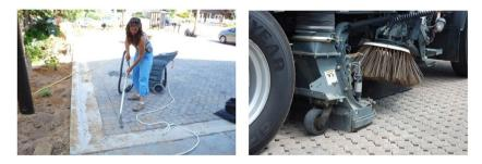
Figure 11. Small-scale (left) and industrial-sized (right) vacuuming of permeable pavement applications.
