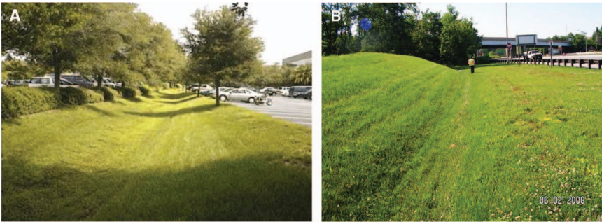
Figure 4-1. Examples of dry swales.
