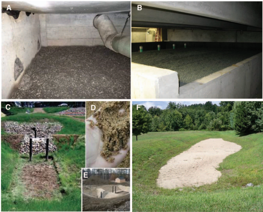
Figure 4-11. A: Filter chamber of underground sand filter contained in Towson University parking garage; B: Filter media chamber and bypass pipe; C, D, E: surface sand filter from University of New Hampshire; F: exposed surface sand filter, Montgomery County, Maryland Department of Environmental Protection.
