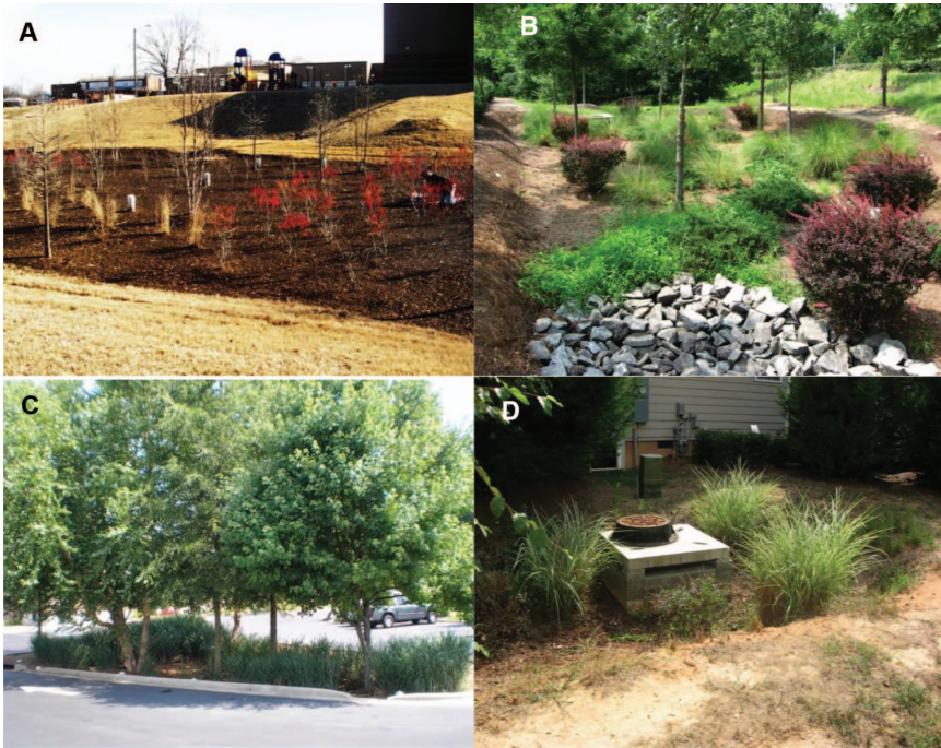
Figure 4-7. Example of rain garden facilities: A: Recently constructed facility at an elementary school; B: bioretention treating rooftop and parking lot runoff; C: bioretention facility in parking lot island; D: small rain garden in residential setting.
