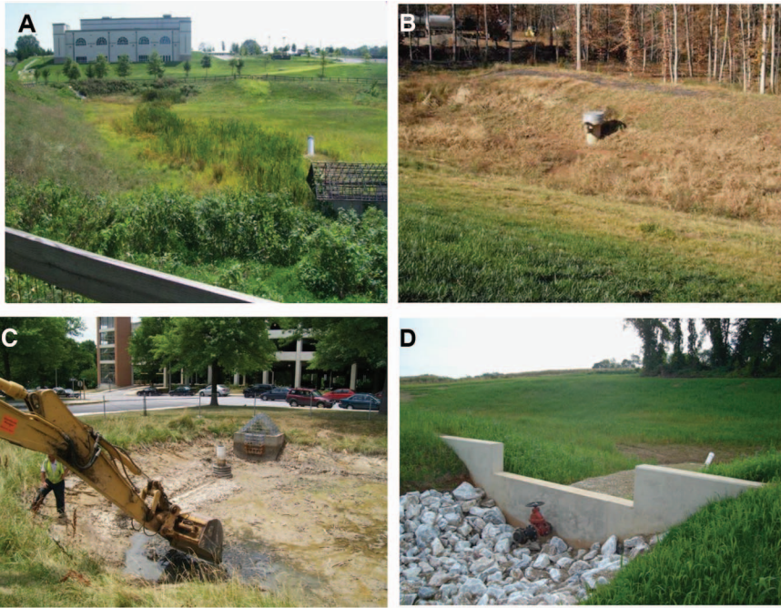
Figure 4-14. Extended detention basin with control structures. (A, B) Dry pond with control structure. (C) Extended detention pond undergoing rehabilitative maintenance. (D) Weir wall outlet structure.
