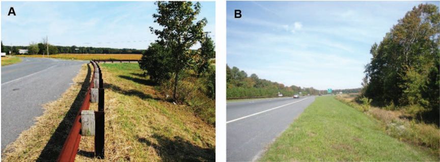
Figure 4-3. Examples of filter strips.
