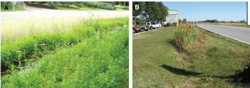
Figure 4-2. Examples of wet swales.
