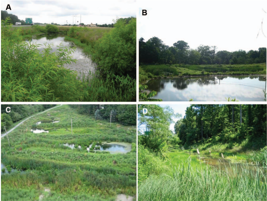
Figure 4-12. Example of wet ponds (A, B) and stormwater wetlands (C, D).
