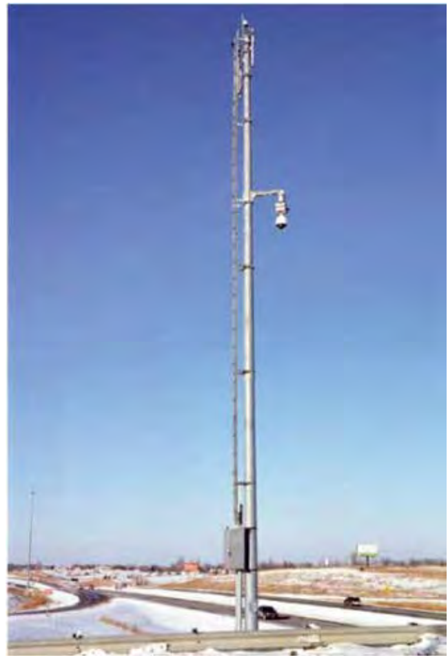
FIGURE 4 RWIS (Courtesy: Kansas DOT).
