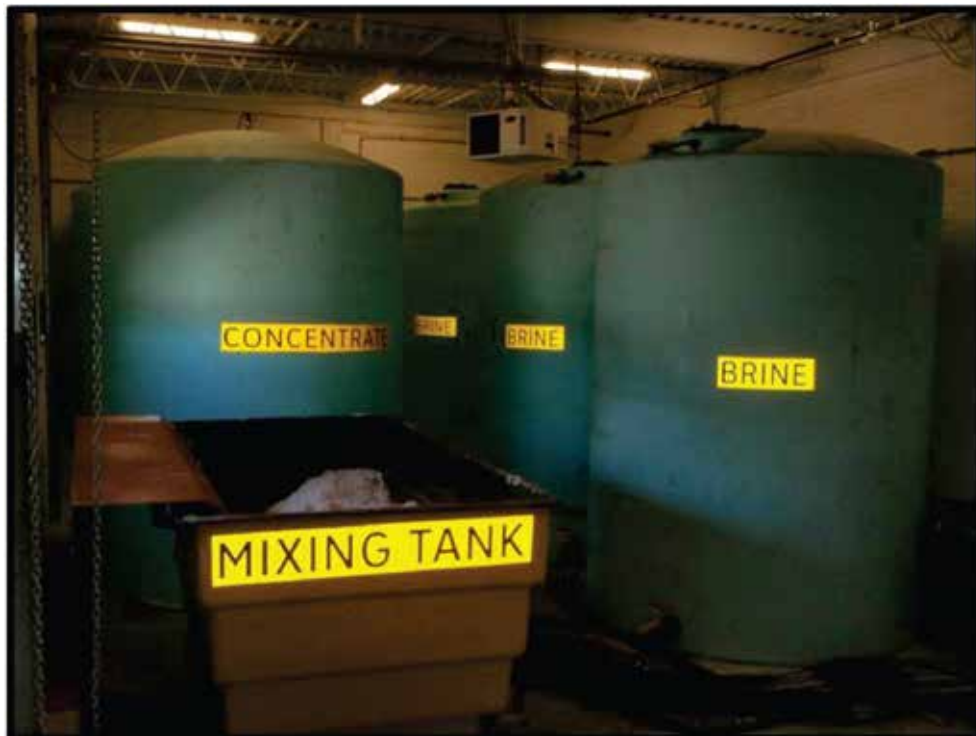
FIGURE B5 The interior of a brine making facility which houses six 5,000-gallon storage tanks, a mixing vessel that holds up to 3 tons of rock salt, and a valve control panel ( Courtesy: City of Toronto ).
