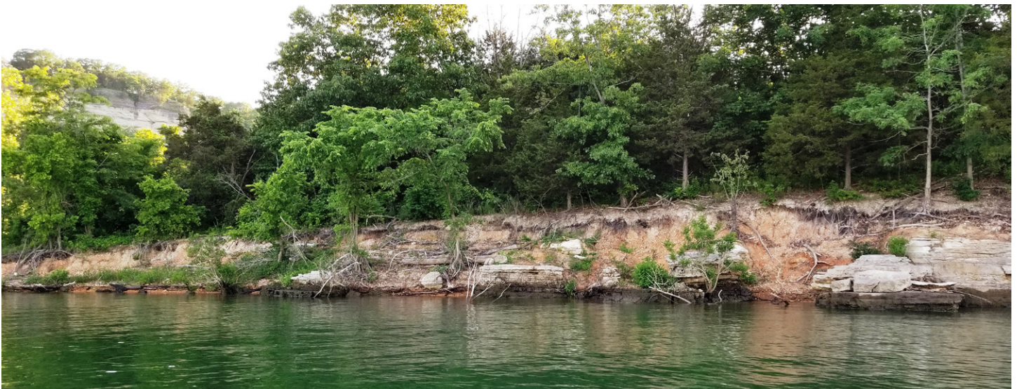
Shoreline erosion at Table Rock Lake.
