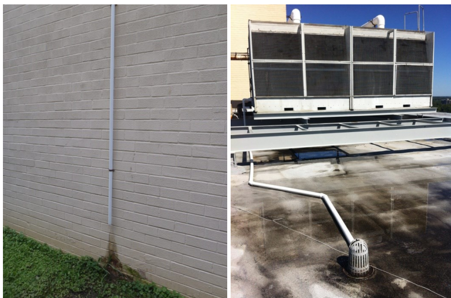
Figure 5. Sample point (left) and cooling tower discharge to roof drain of the same building (right). The roof drains are probably connected to the MS4 underground.
