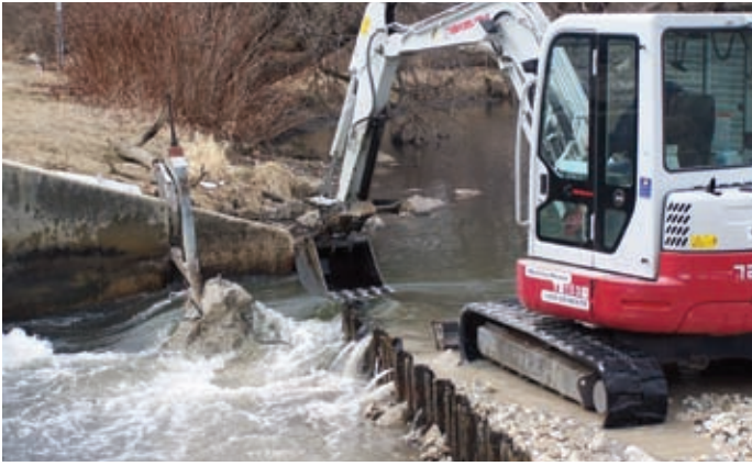
Figure 5. Removal of the Churchill Woods dam gets underway.
