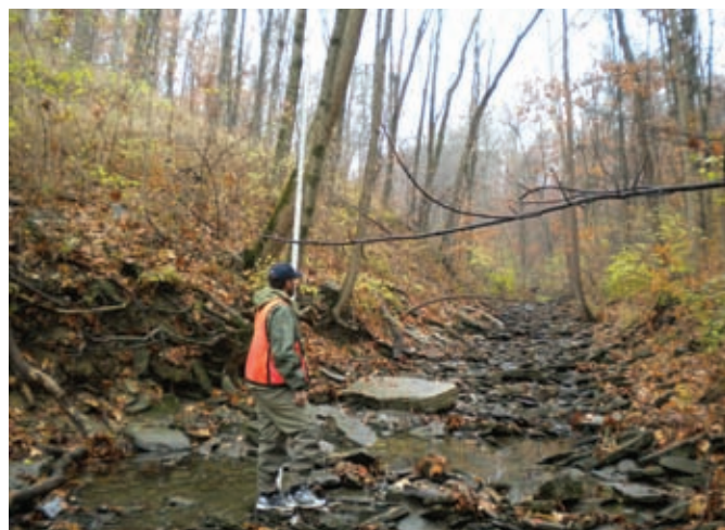
Figure 3. Looking upstream at the DA2-DS site in Pleasant Run (note failure of left bank).
