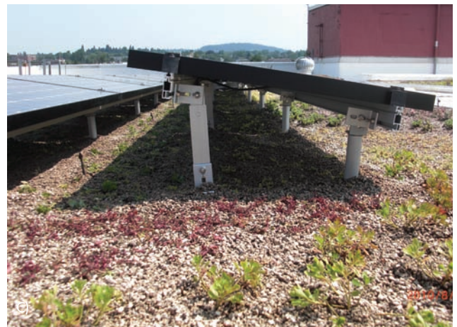
Figure 1. Ecoroof examples include a backyard community effort (A), an ecoroof overlooking the Willamette River (B) and inclusion of solar panels (C). Photos courtesy of the City of Portland, Bureau of Environmental Services.
