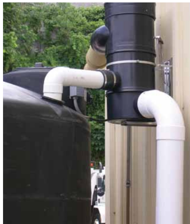
Figure 2. This vortex filter is an example of a pretreatment device for rainwater harvesting. The vortex filter diverts the first amount of rainfall, which tends to have a lot of solids and vegetative debris. Vortex filters come in different sizes based on efficiency curves for rooftop area treated and rainfall intensity. Photo courtesy of: Rainwater Management Solutions, Inc.
